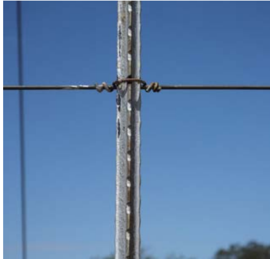
09 A close-up image of an electric fence with wire threaded through a Y-standard and secured with an additional coil of wire by Agri-Wire (EDMS).
