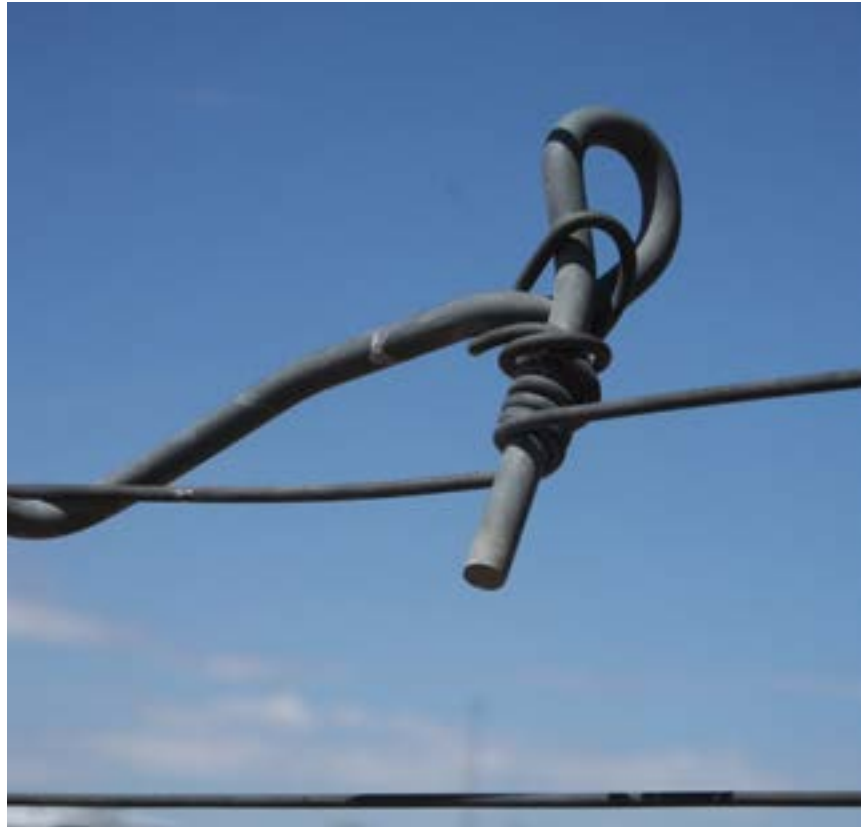
05 Loops of wire around an eye bolt securing a fence in place
